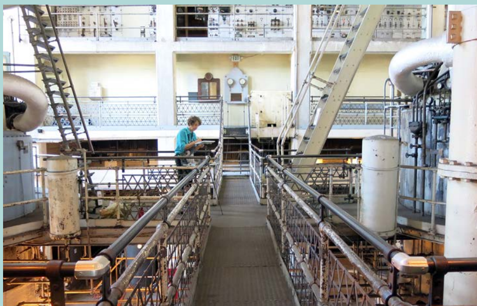
Georgetown Steam Plant
