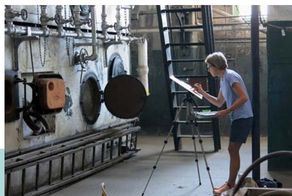
Georgetown Steam Plant
